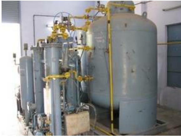
NITROGEN, OXYGEN and SUCTION TANK ROOM
